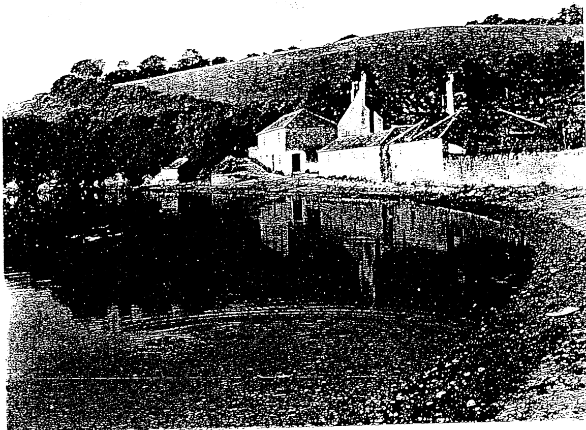
NEARLY SHOWING Galimpton Mill. Lot 4 ACCOMMODATION ROAD S. 437 AROUND FORESHORE 1944 THEN O.S. 366
